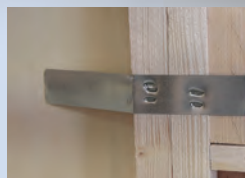
Hurricane Straps Add Strength and Safety
